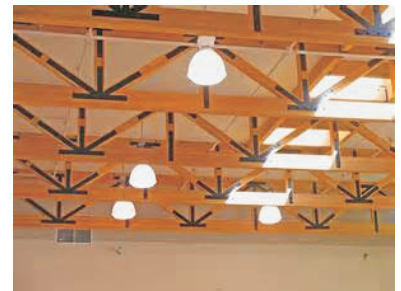
EXAMPLE OF A WEB JOIN
