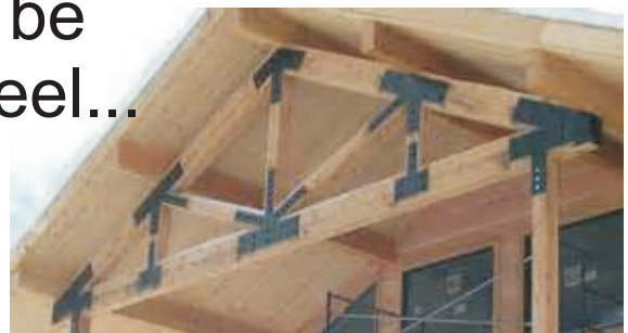
EXAMPLE OF A WEB JOIN
